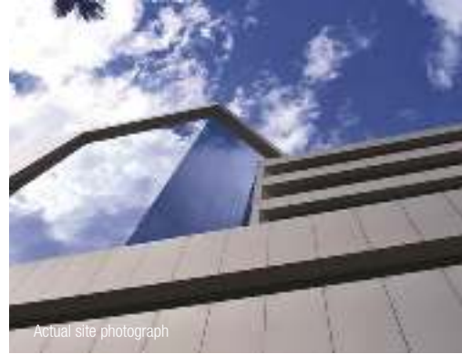
GODREJ CASTLEMAINE BUND GARDEN, PUNE
