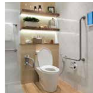
HAND RAILING IN ONE TOILET
