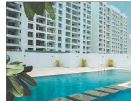
GODREJ HORIZON NIBM ANNEX, PUNE Completed in 2015
